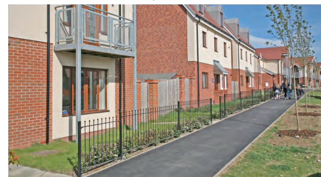
An example of a typical garden depth with railings that clearly define private space from public space.
